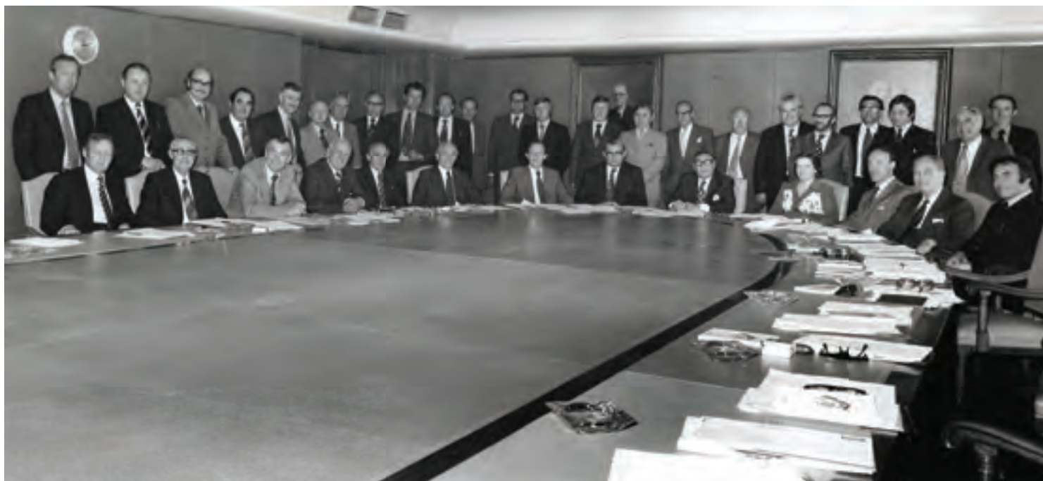
A Wimpey board meeting at headquarters in London the mid-1970s. Bill Lowry is standing, second from left.
